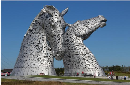
A contract was awarded in May 2012. SH Structures used 3D design software which enabled them to consider how to modularise structures which was essential for fabrication and in turn helped with the planning the lifting and turning of units, and their transportation and site erection. Tim paid tribute to the 40 skilled platers and welders in the company who were instrumental in building the modules and
